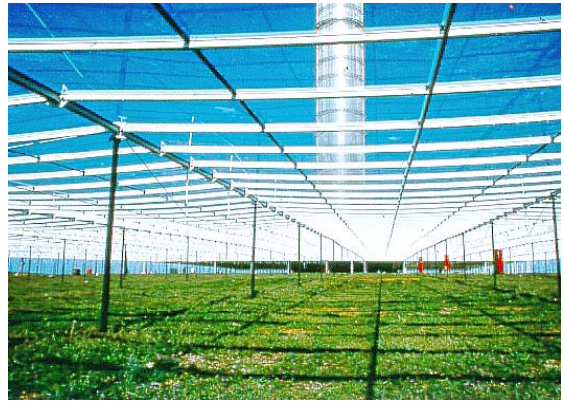
Figure 6. Glass roof of the prototype plant at Manzanares, Spain.
