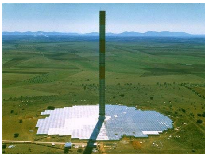
Figure 4. Prototype of the solar tower prototype plant at Manzanares, Spain
