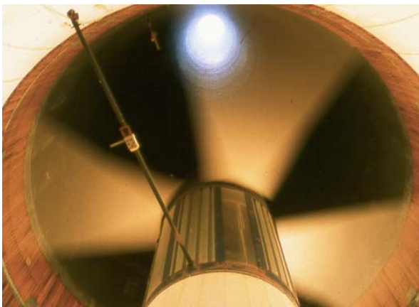
Figure 5. Turbine of the prototype plant
